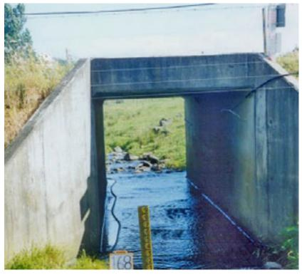
Figure 9 Single box culvert
