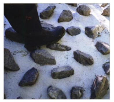
Figure 11 Rocks can be cemented into the base of waterway crossings and/or to the aprons of culverts to ensure that there are areas of low water velocity available to aid fish passage and sediment which is appropriates for invertebrates is retained within the structure
