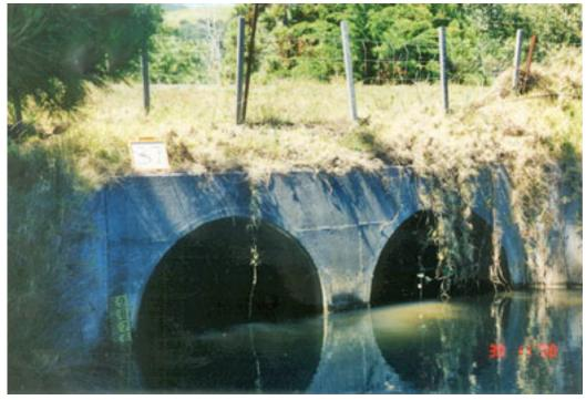
Figure 7 Typical multi-barrel circular culvert
