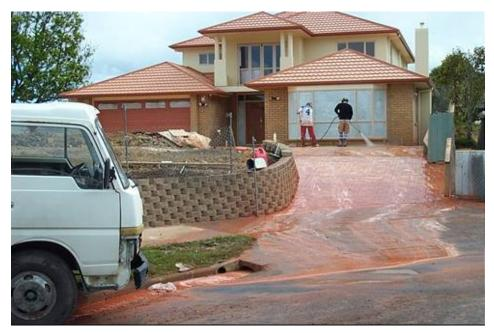
Photo 1: Stormwater being contaminated from waterblasting a driveway
