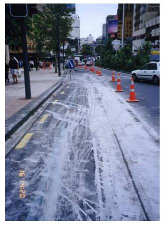
Photo 2: Contaminants from concrete cutting running into stormwater systems
