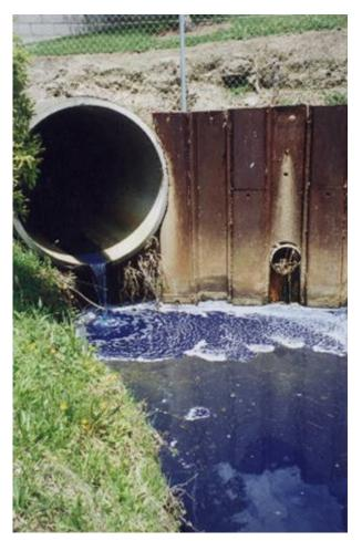
Photo 3: Release of contaminants to stormwater from a paint spill
